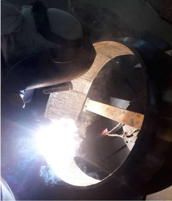
SMAW Overlay on Flange ID
