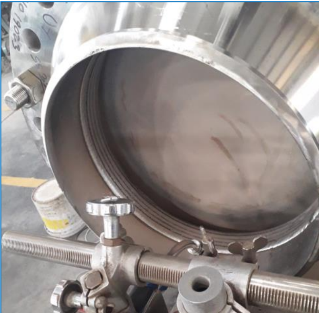
Automated FCAW on Flange ID
